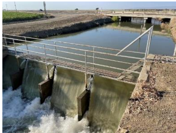
Figure 50. Colony Main Canal headworks measurement weir, looking upstream; not shown is a turnout to the right
