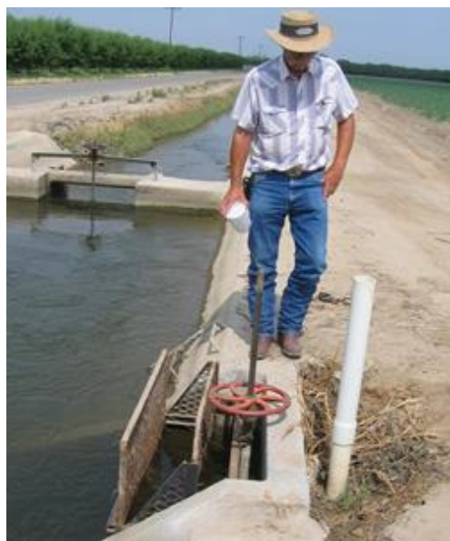
Figure 10. This stilling well is properly located, but it has too small a diameter. The operator also needs to know the elevation difference between the top of the stilling well and the gate frame, which requires an extra computation to determine the difference in head across the gate.
