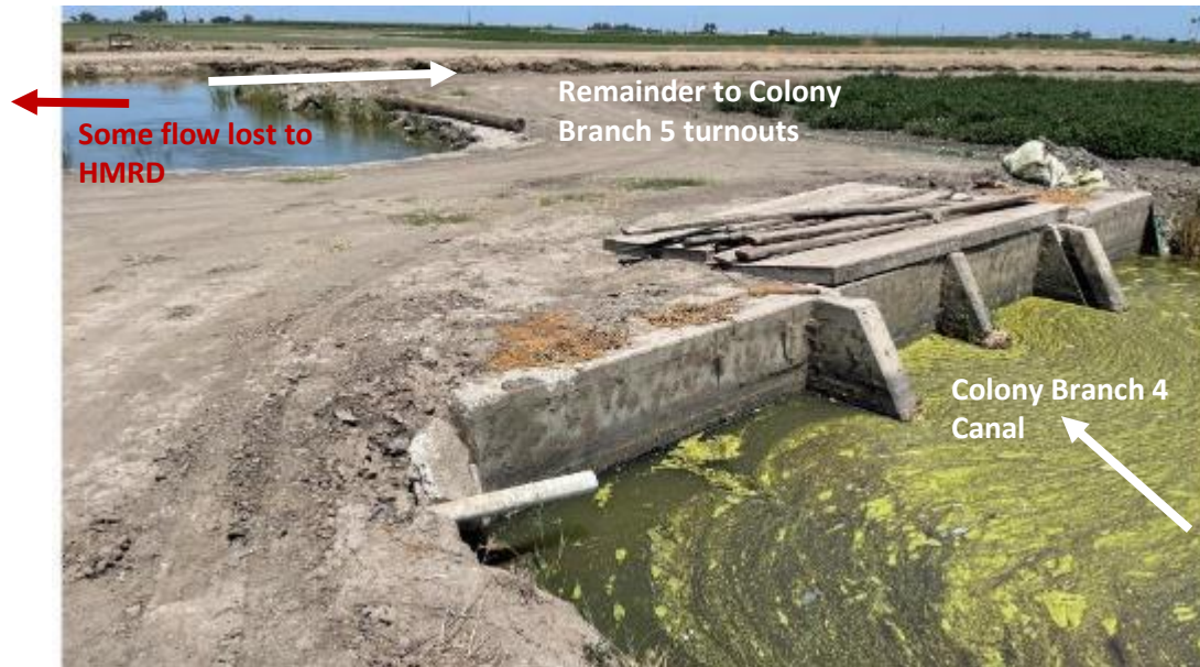
Figure 90. Existing Colony Branch 4 spill weir structure and downstream convergence with Colony Branch 5. Note that spill flow is lost to HMRD and is unrecoverable.
