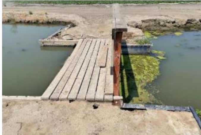
Figure 106. Existing wood and steel weir, the second check along Shafter Ditch
