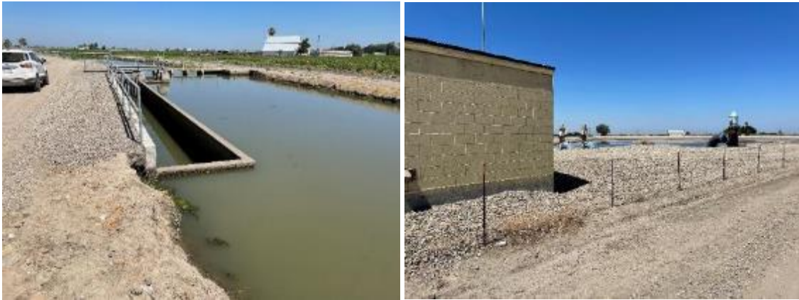
Figure 57. Existing Colony Main Reservoir inlet weir (left) located at an upstream check; Inlet and outlet pumps (right) at reservoir bank
