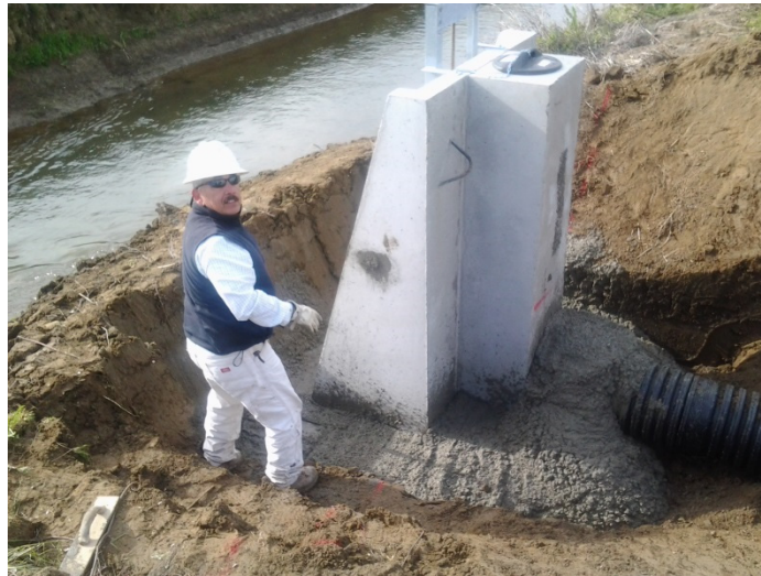
Figure 15. Installation of GCID metergate
