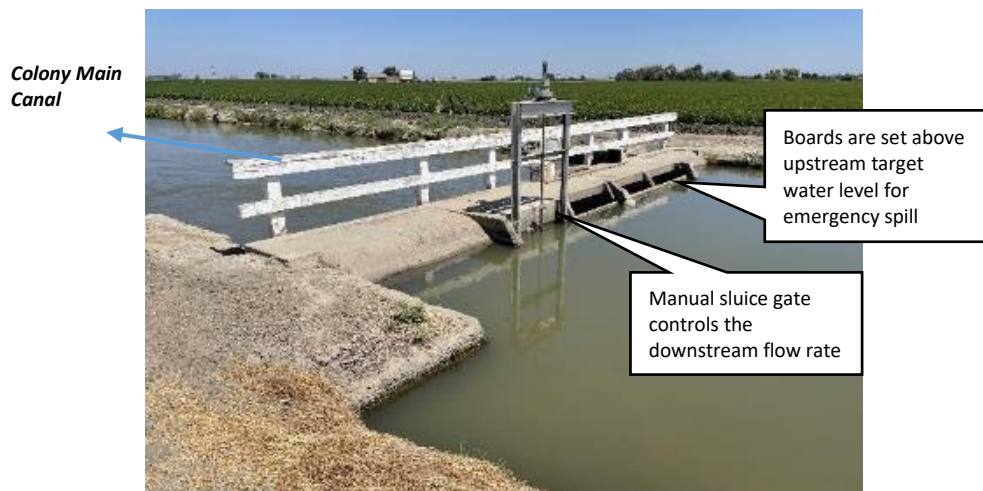
Figure 58. Colony Main Canal 13.213 structure just downstream of the existing buffer reservoir, looking downstream
