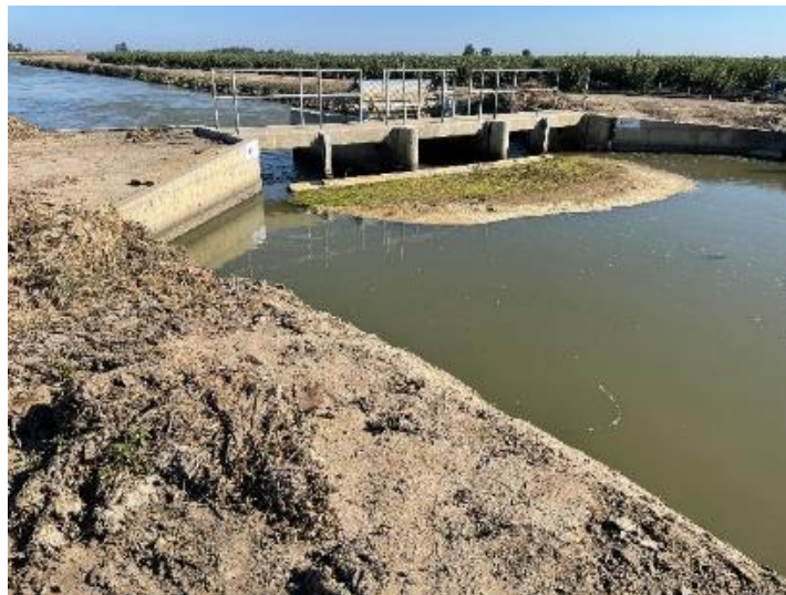
Figure 52. Unique Colony Main Canal 3.265 check structure; a combination of flashboards and a manual radial gate
