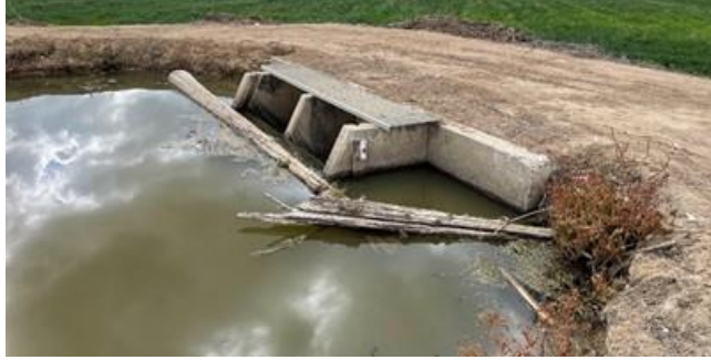
Figure 13. Existing flashboard structure located at the tail end of the Sullivan Extension open channel
