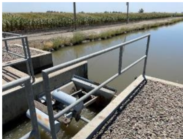
Figure 101. Existing AMIL gate, installed at the Machado Weir, looking upstream
