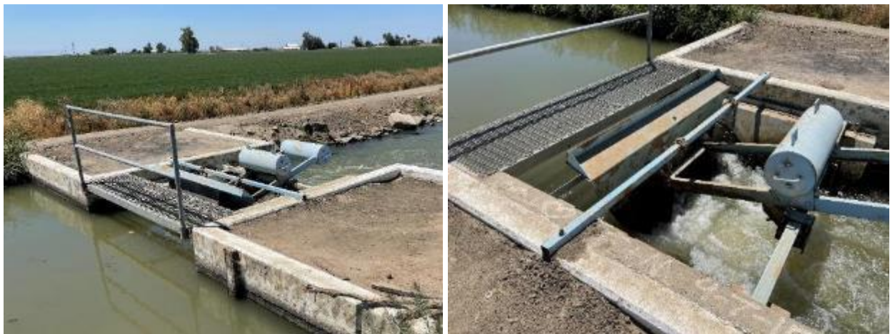
Figure 79. Two views of the existing AMIL gate check along Colony Branch 3 at station 82+50
