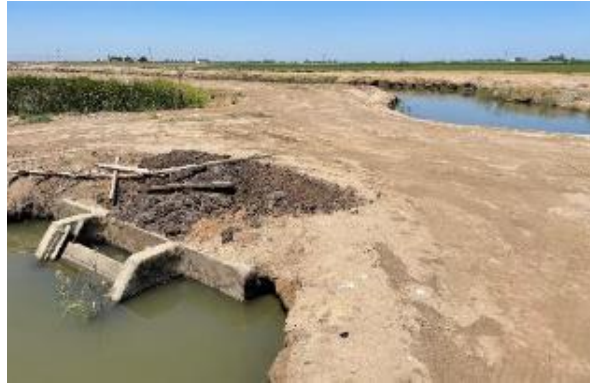
Figure 102. Existing Branch 5 Canal spill structure; the new HMRD spill flow monitoring site is just downstream; existing top of concrete elevation = ~102.5'
