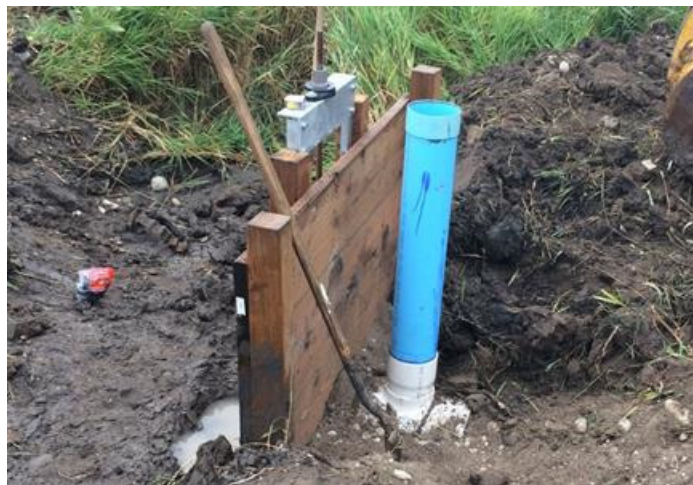
Figure 8. Stilling well installed on an existing discharge pipe. It is constructed of PVC pipe that is too thin for long life, but it serves as an example of the correct diameter, position, and height.
