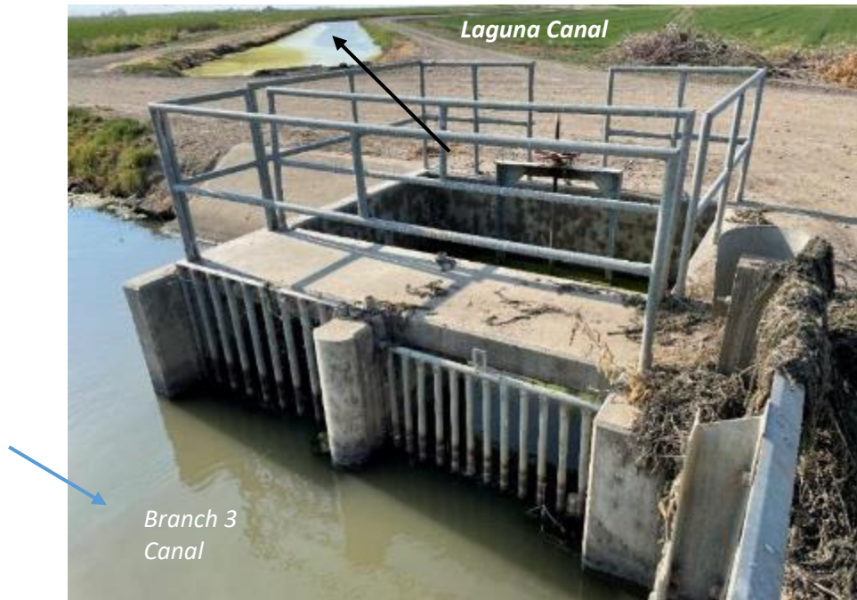
Figure 20. Continuation of the Laguna Canal, looking downstream (north); the gate may be used to set a target flow rate
