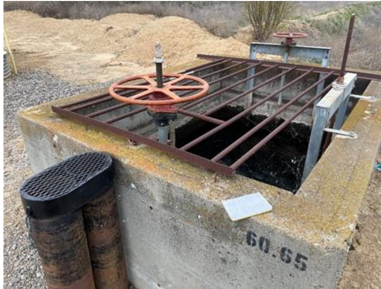
Figure 26. DMC 60.65 distribution box; the gate supplying CCID is in the foreground
