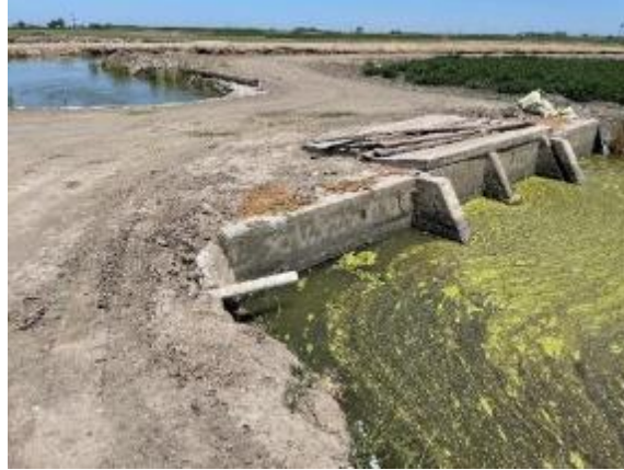
Figure 96. Branch 4 Canal tail end spill weir structure; set board crest elevation to 102.3' (top of existing concrete at 104.2')
