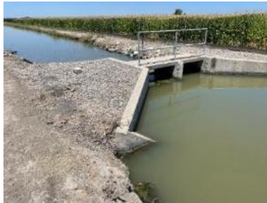
Figure 100. Existing first flashboard check along Branch 5 canal; looking downstream
