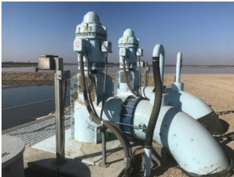
Figure 40. Poso Reservoir pumps, with compacted native soil and rip-rap lined banks visible in the background
