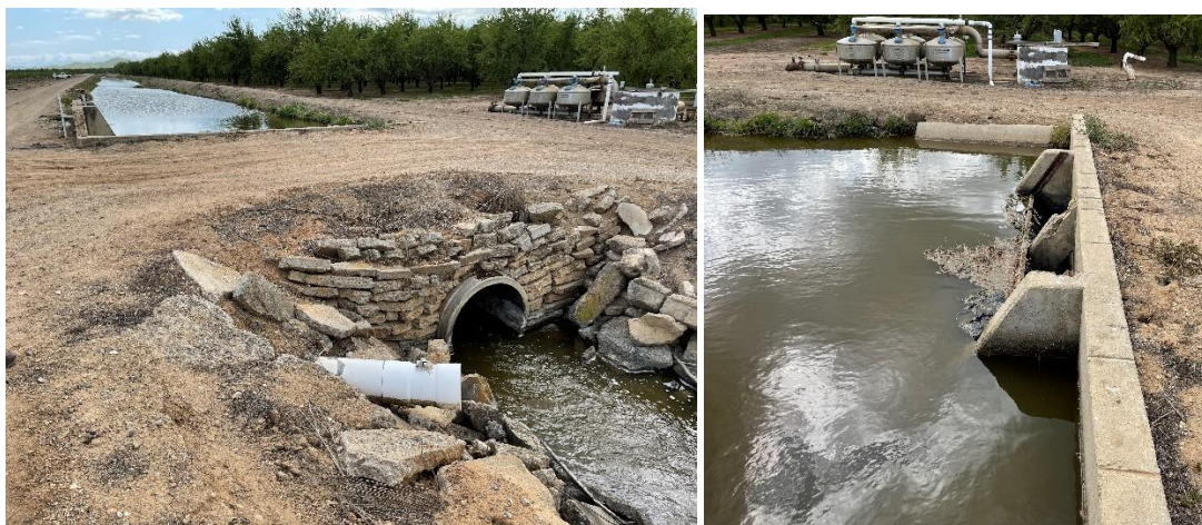
Figure 11. Existing conditions at the first flashboard check, looking upstream (see left image) and the flashboard structure (right)
