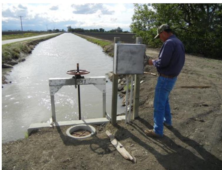
Figure 12. Large diameter stilling well, with cover to minimize having it fill with dirt from the road. Strong concrete, with the rim of the stilling well at the same elevation as the bulkhead top.
