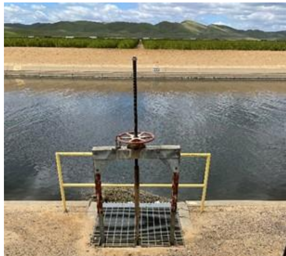
Figure 25. DMC 60.65 36" canal gate; left open most of the time
