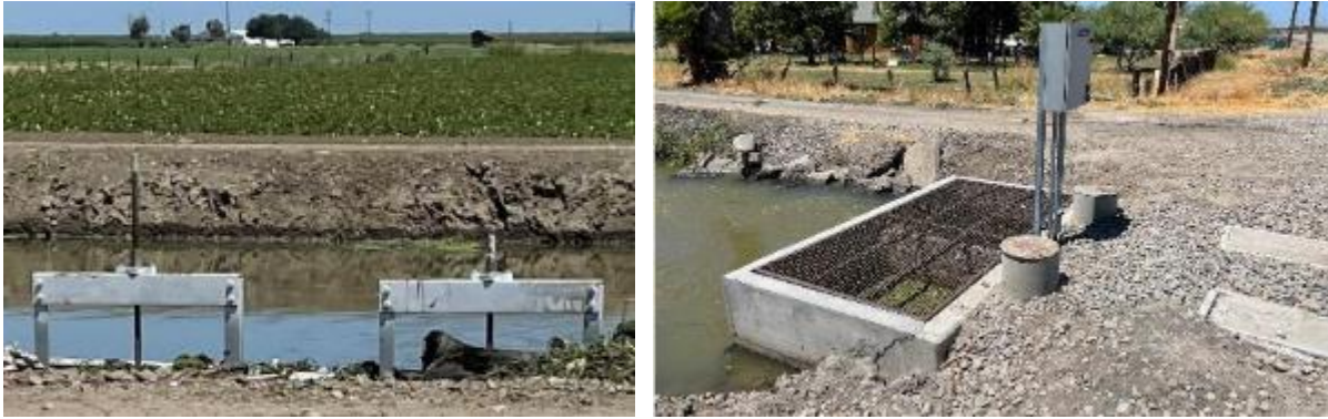
Figure 88. Colony Branch 4 headworks, with 30" two canal gates (on left, looking upstream at the Colony Main Canal) and individual acoustic Doppler flow meters (on right) at the culvert discharge
