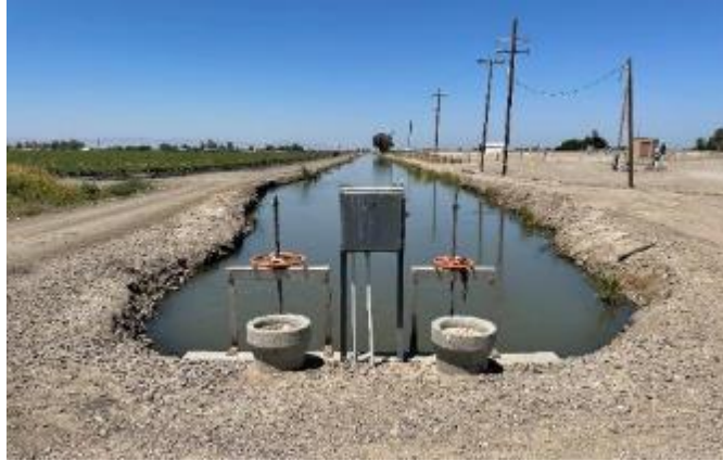
Figure 99. Existing 30" Branch 5 Canal headworks gates, fitted with individual flow meters, looking downstream
