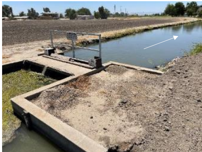
Figure 89. Branch 4 Canal 1.125 check, an existing flashboard structure, looking downstream; note the failing concrete walkway
