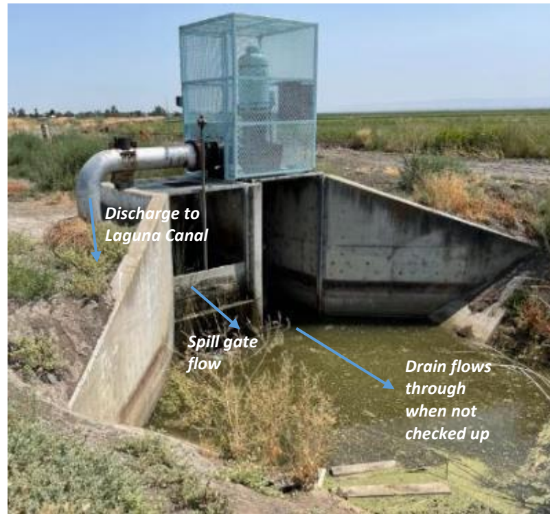
Figure 32. Existing Shain Drain pump station and Laguna Canal spill structure at station 77+61
