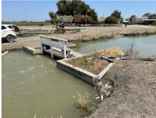
Figure 16. Laguna Canal 2.913 weir board check structure; similar throughout with a few exceptions
