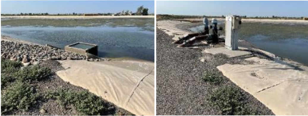
Figure 18. Existing Laguna Reservoir inlet weir (left) and outlet pumps (right)
