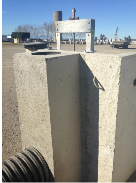
Figure 13. GCID metergate at Briggs
