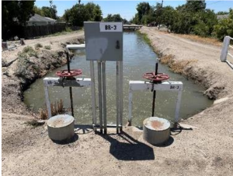
Figure 78. Existing Branch 3 Headworks gates, looking downstream
