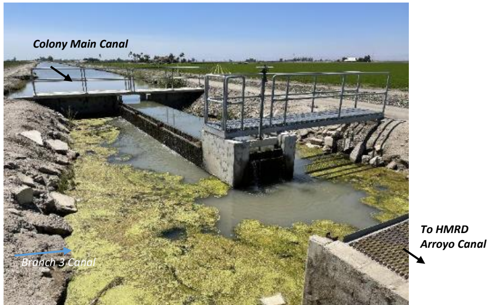
Figure 59. Terminus of Colony Main Canal just upstream of HMRD Arroyo Canal
