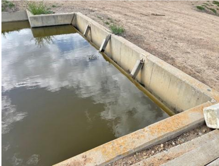
Figure 15. Existing flashboard check at Flashboard Structure A (FB A).
