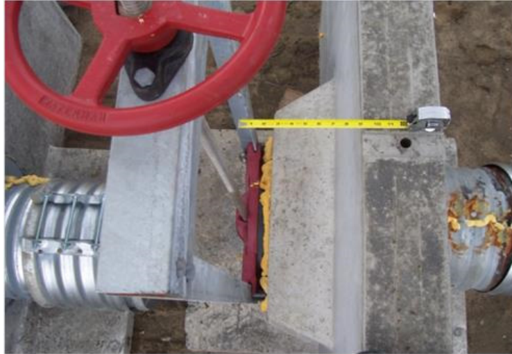
Figure 7. Stilling well is located the correct distance downstream of the gate, but is so small that there will be tremendous surging (up/down movement), and operators cannot see the water surface
