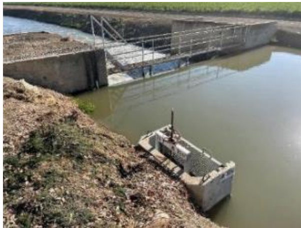
Figure 49. Colony Main Canal headworks measurement weir, looking downstream
