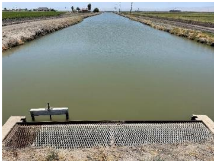
Figure 43. Laguna Canal tail end, looking upstream. Weir to be removed and culvert to be enlarged.
