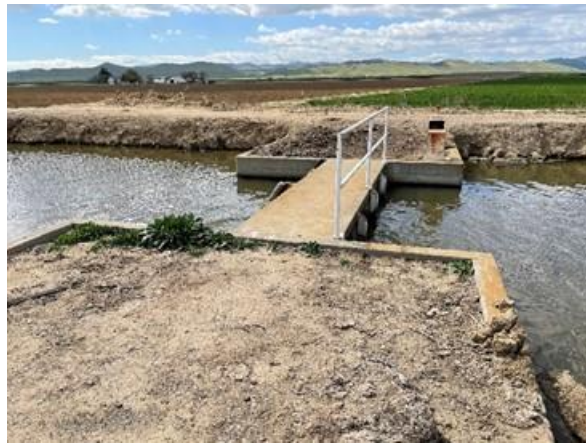
Figure 18. Abandoned flashboard structure just downstream of Garzas Creek – to be demolished
