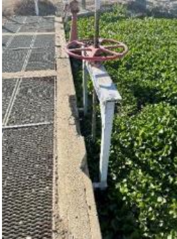
Figure 48. Colony Main Canal flow control gates; note the different types of gates and the failing concrete
