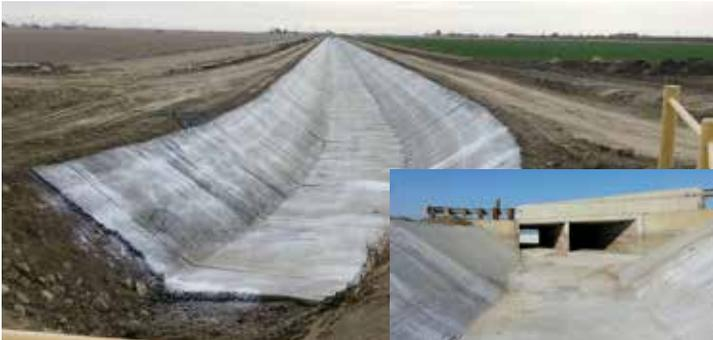
*Second Phase of Firebaugh Canal's 1st Lift Canal Lining Project included lining some 2 miles of canal for improved efficiency, maintenance and delivery.*
