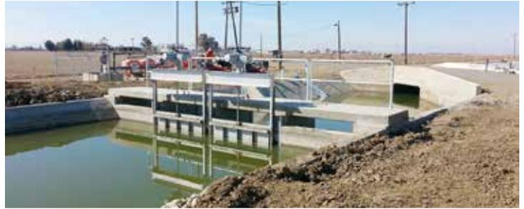
*The project also included construction of a new automated check structure that will be operated through the District's SCADA system.*
