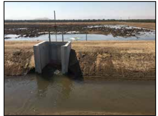
Ponding efforts at Orestimba Creek Recharge and Recovery Project.
